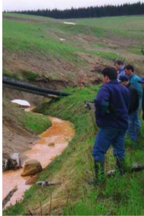
The covered waste rock tip with collection of seepage (Equility Silver Mine, B.C., Canada).
