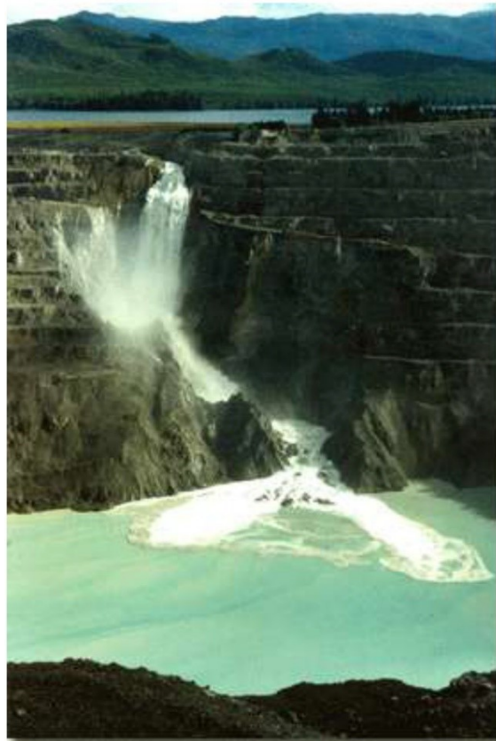
Island Copper Mine, British Columbia. Filling of the open pit mine with seawater from the Rupert Inlet fjord after mining was phased out in 1995. The world's highest seawater waterfall!
