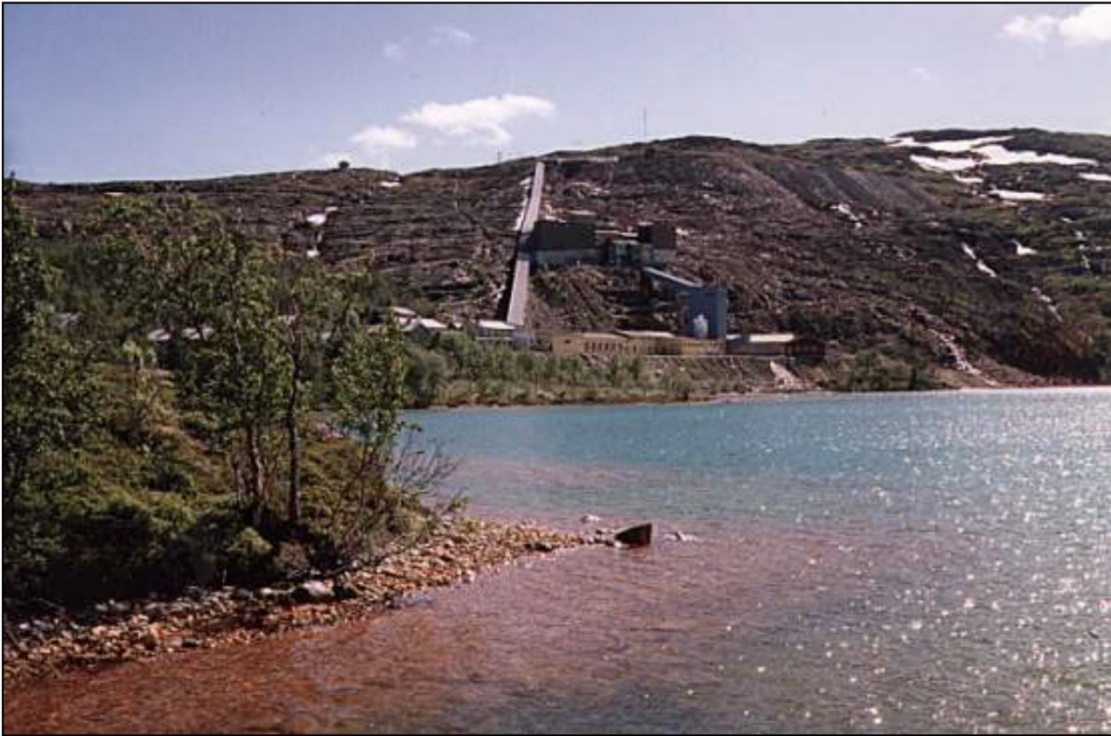
Mine in Skorovatn lake with the waste rock tip. Photo: Rolf Tore Arnesen, 1988.
