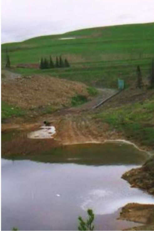
The covered waste rock tip with collection of seepage (Equility Silver Mine, B.C., Canada).
